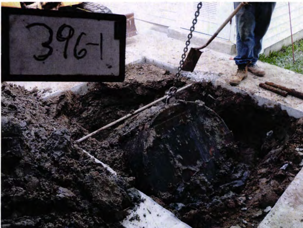
Picture 2: UST 396Acorn-1 being removed.
