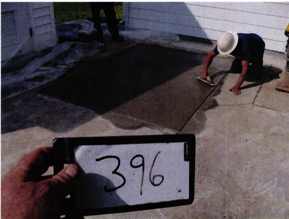
Picture 4: Tank removal finishing touches.
