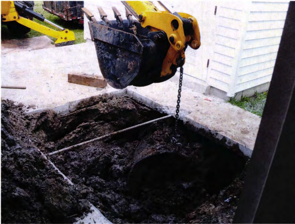
Picture 3: Removal of UST 396Acorn-2.
